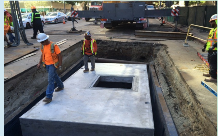
Vault installation on 5 th /Flower intersection
