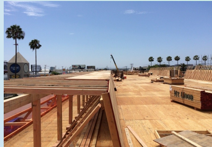
AVIATION/CENTURY STATION – Bridge falsework for concrete pour
