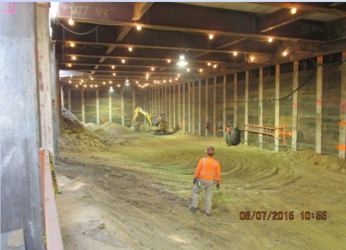
LEIMERT PARK STATION – Excavation and lagging
