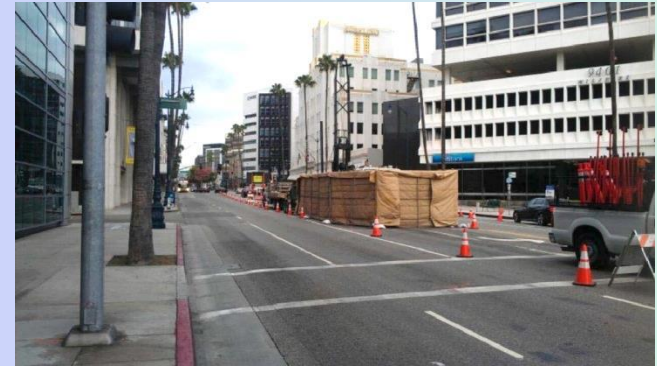
Geotechnical Drilling on Wilshire at Reeves
