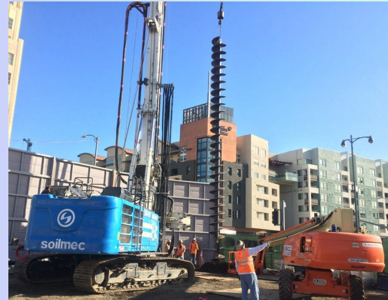
Pile Installation Activities at the Wilshire/La Brea Station
