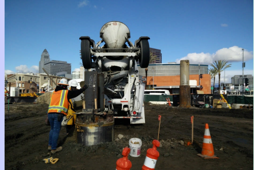
Soldier Pile Installation at 1 st /Central Station
