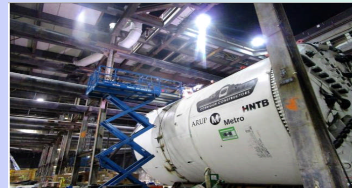
Start of TBM assembly in Expo/Crenshaw Station
