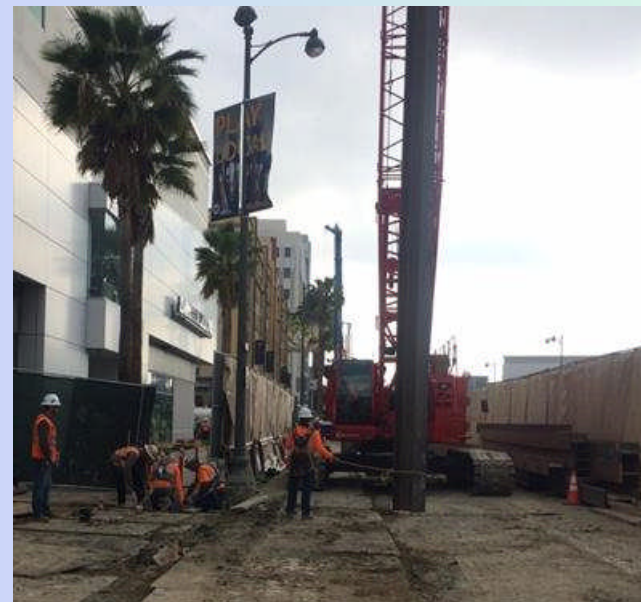
C1045 Contractor Installing Pile at Wilshire/La Brea Station
