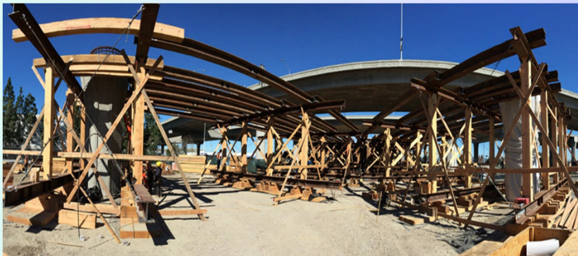
Crenshaw tie-in with Green line falsework construction
