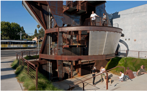
Figure 12 EOM Samitaur Tower
