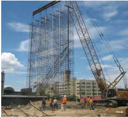
Figure 3-15: Steel Reinforcement Cage for Slurry Wall
