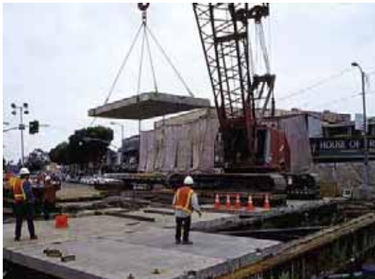
Figure 3-4: Installation of Decking (1 of 2)
