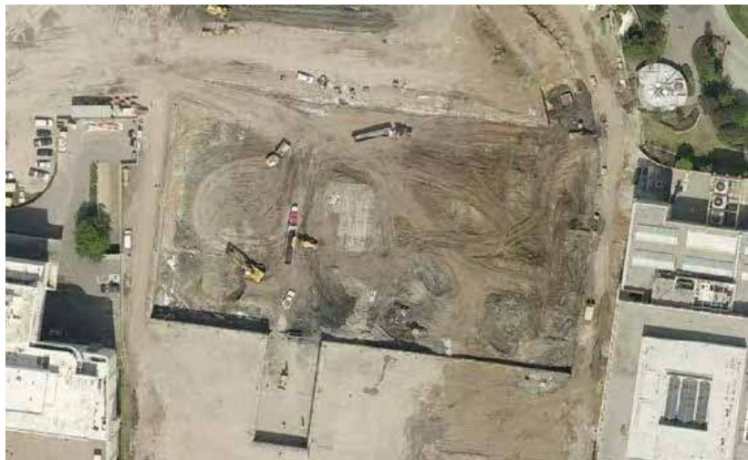
Figure 4-17: Aerial View of Project 23 Excavation with Dark Tar Seeps
