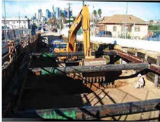
Figure 4-12: Hydraulic Excavator between Struts
