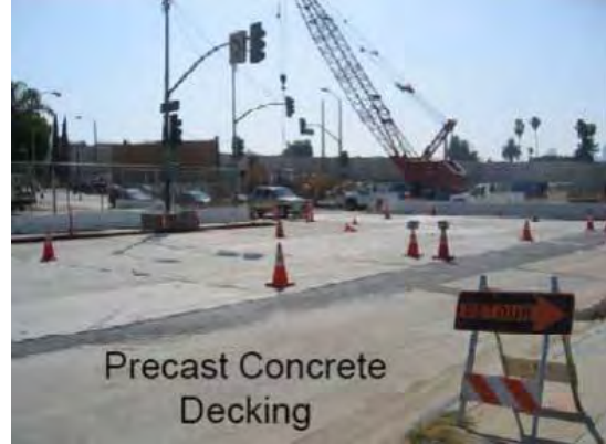
Figure 3-4 Precast Concrete Decking
