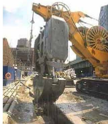
Figure 3-15: Clamshell Digger for Slurry Wall Construction
