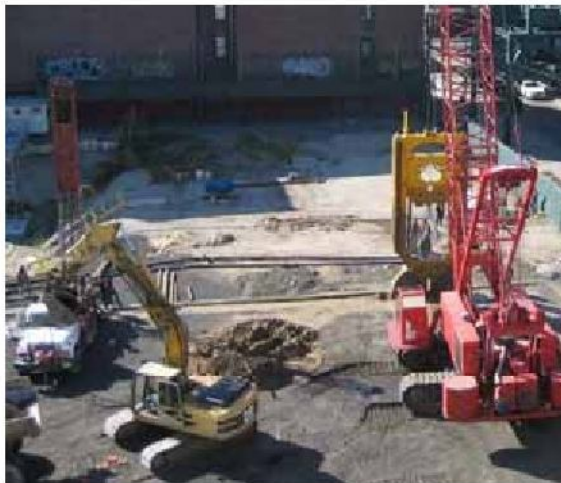
Figure 3-14: Slurry Wall Construction Equipment
