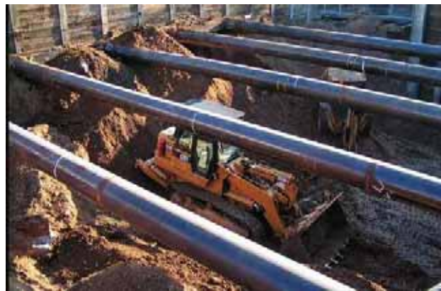
Figure 4-13: Track Loader beneath Struts
