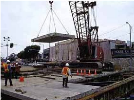
Figure 3-4: Installation of Decking (1 of 2)
