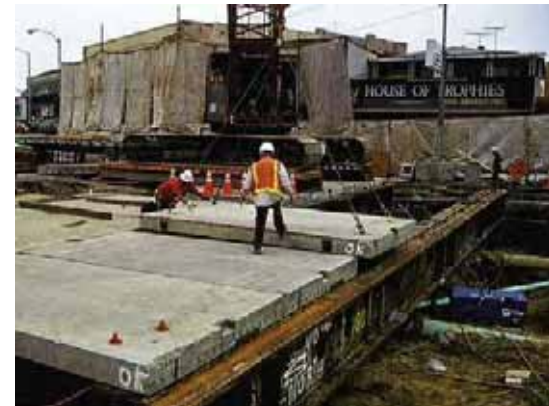
Figure 3-5: Installation of Decking (2 of 2)
