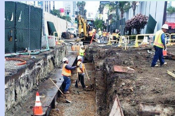
Wilshire/La Brea Station – Preparation for Deck Beams
