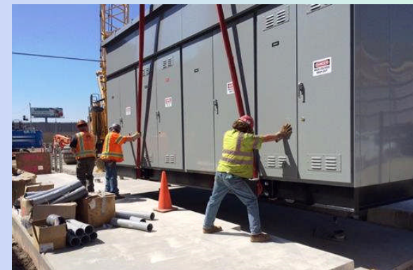
Electrical Metering Switchgear for Tunnel Operations
