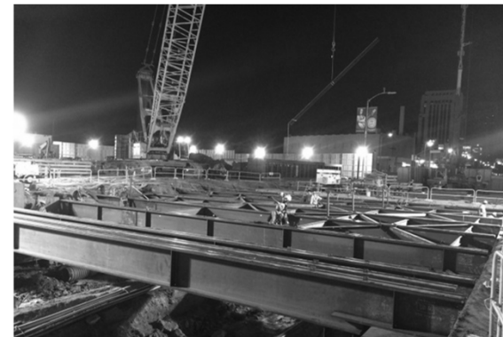
Installation of Deck Beams on Wilshire Blvd.
