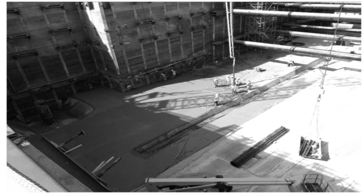
Pouring mud mat at 1 st /Central Station
