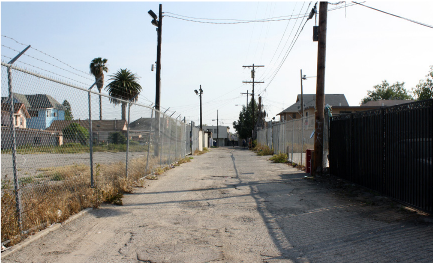
Existing Alley Condition, 2016
