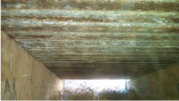
Picture 5: The inside of one of the top 3 Priority "Rail-Top" Bridges on the Valley Subdivision
