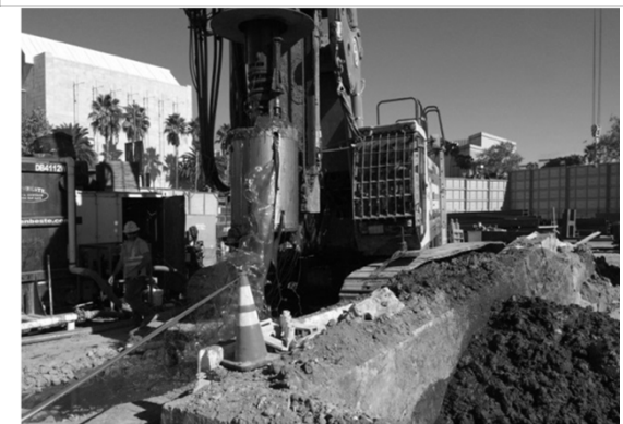
Drilling Piles at Ogden Yard
