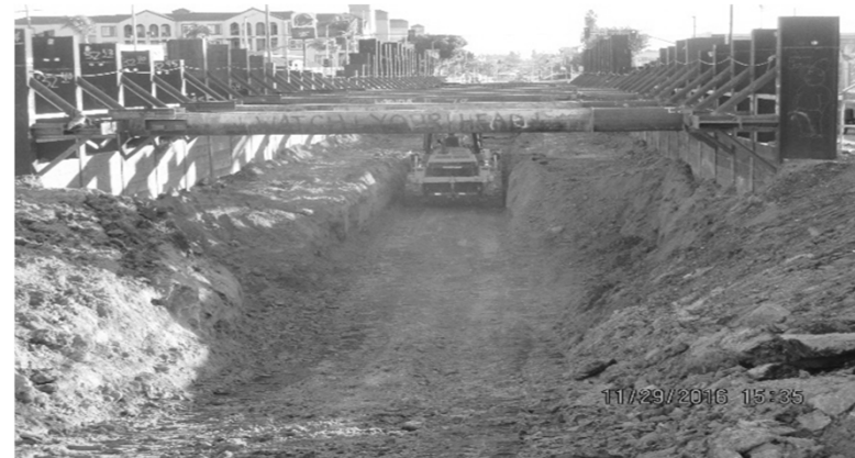
Excavation continues for underground structure on Crenshaw Blvd
