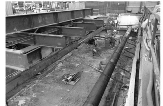
Installing Strut at Wilshire/La Brea Station
