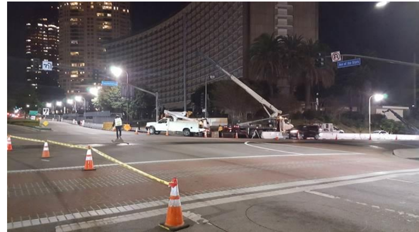
Telecom joint trench construction at Constellation Boulevard
