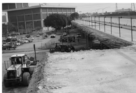
Edge of Deck Removal
