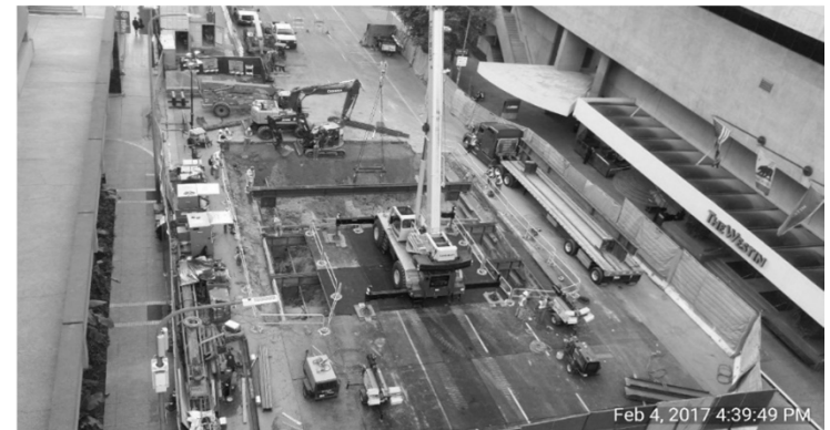
Installation of deck beams on Flower Street
