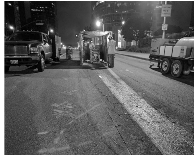
Telecom Joint Trench Construction along Constellation Boulevard
