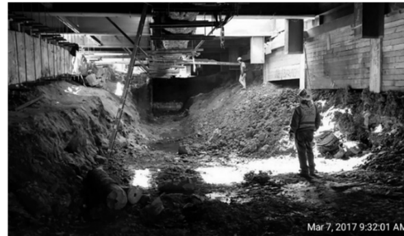
Utility hanging under 2 nd Street decking
