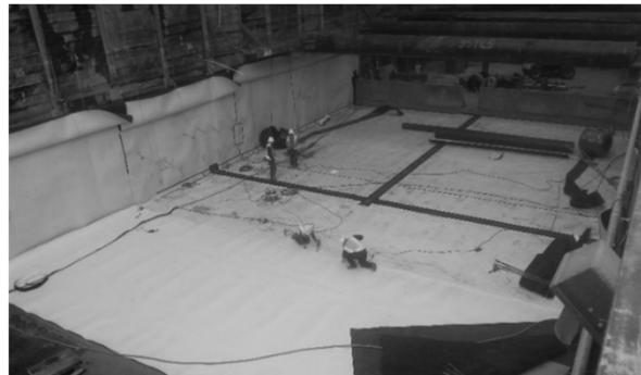
HDPE placement at 2 nd /Hope Station
