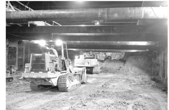
Under Deck Excavation at Wilshire/La Brea Station
