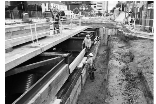
Decking Operation at Wilshire/Fairfax Station
