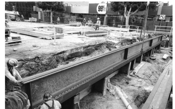
Decking Operation at Wilshire/Fairfax Station
