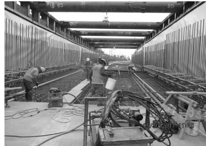
Installation of rebar for UG#4 south of Leimert Park Station.
