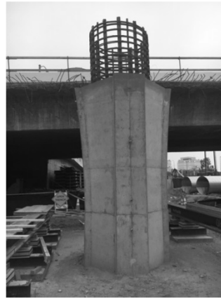
Completed bridge column
