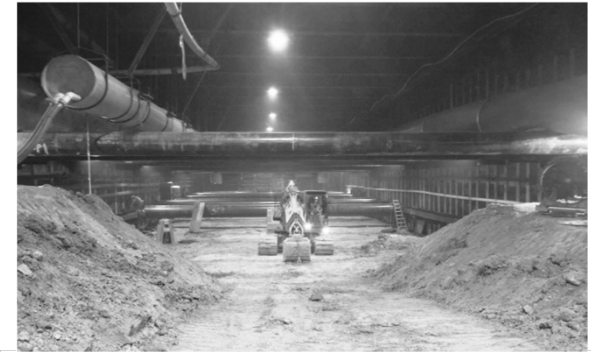
Under Deck Excavation at Wilshire/La Brea Station
