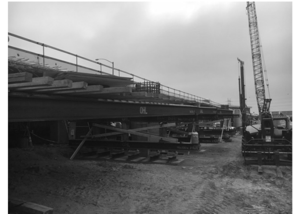
False work on south side
