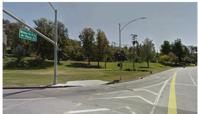
Figure 0-12: Facing South at Workman Mill Road and Peck Road Intersection
