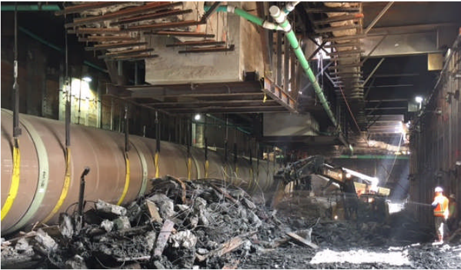
LA County storm drain demolition adjacent to Hobas replacement
