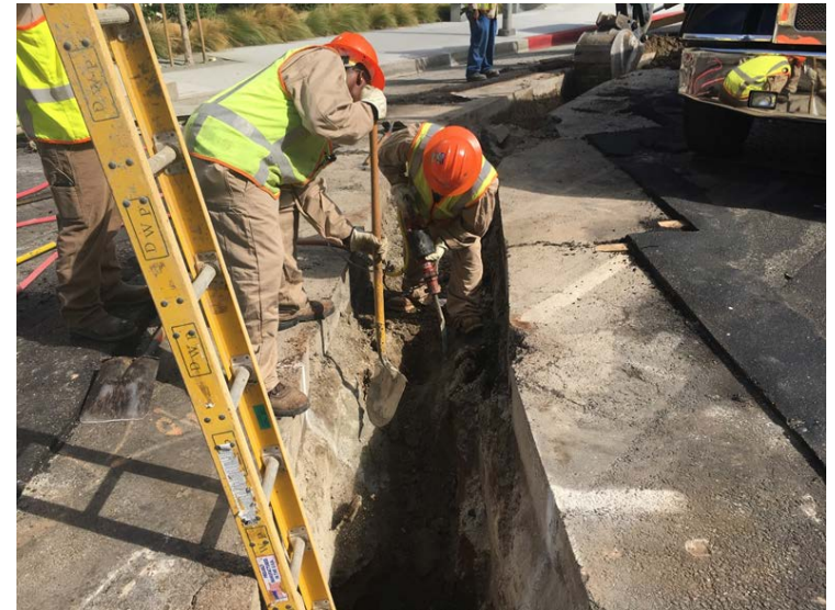
LADWP power relocation work in Century City
