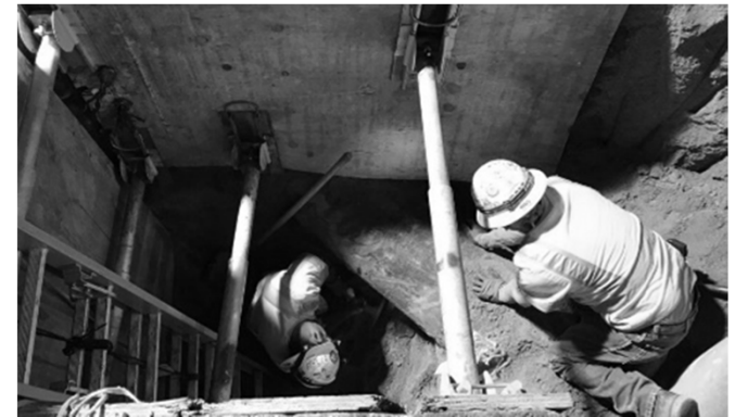
Excavation of 20" waterline on Central Avenue
