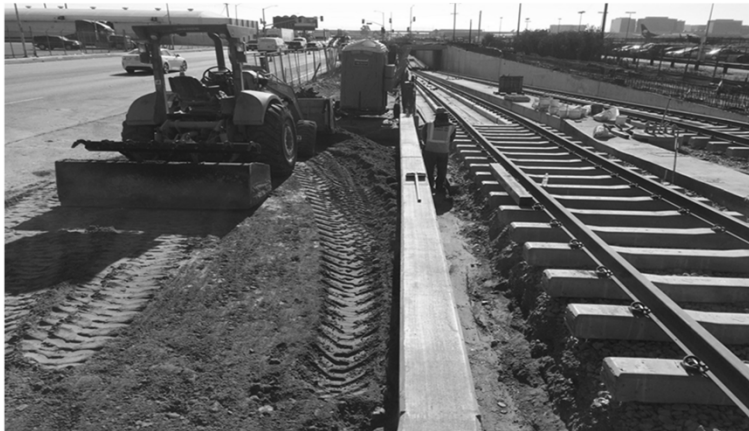
Backfilling continues on main line near LAX Airport runways
