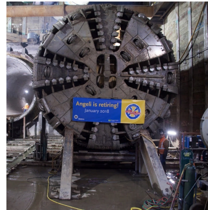
Tunneling completed January 16, 2018
