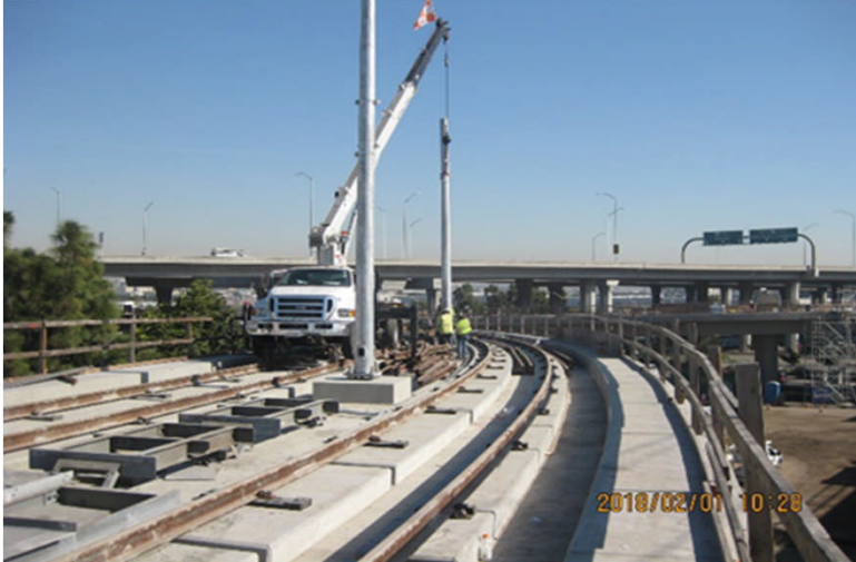
Setting overhead catenary system poles – south end
