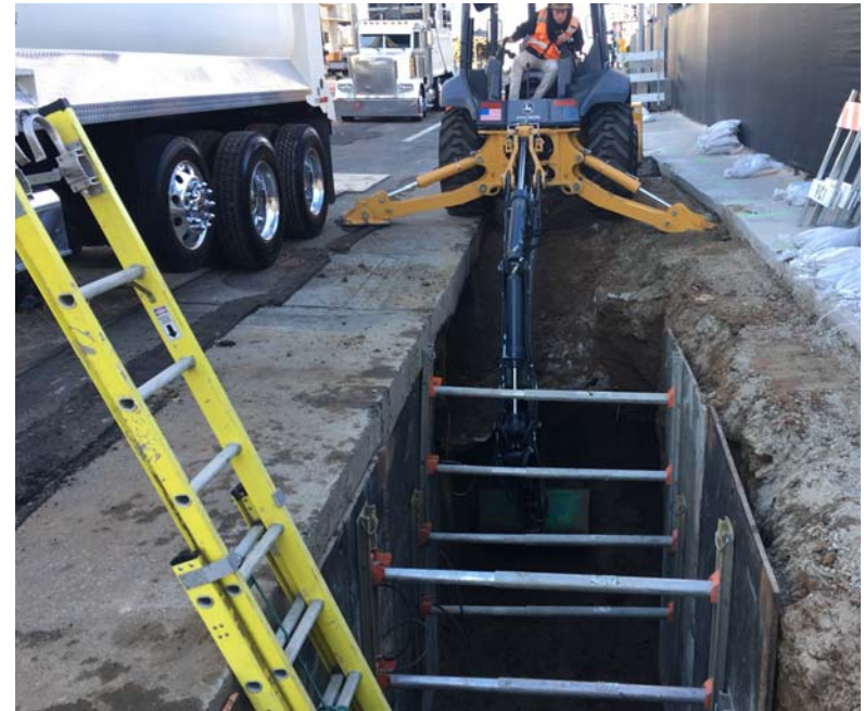
AT&T Conduit Installation in Century City
