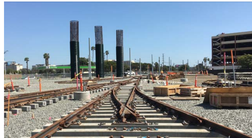
UG #3 Cut-and-cover tunnel – track work plinth construction Southwestern Yard – south yard track leads & APM columns
