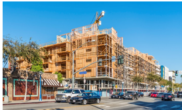
Mixed-use Development – La Brea Ave.
