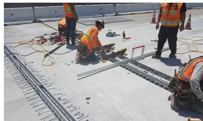
Joint Seal Assembly Install
