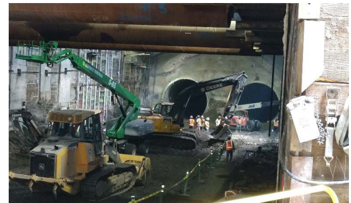
Sequential Excavation Method (SEM) underway at Historic Broadway Station
