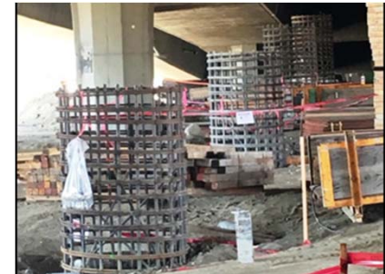
4 Ped OC foundations are incomplete and require only forming and pour
