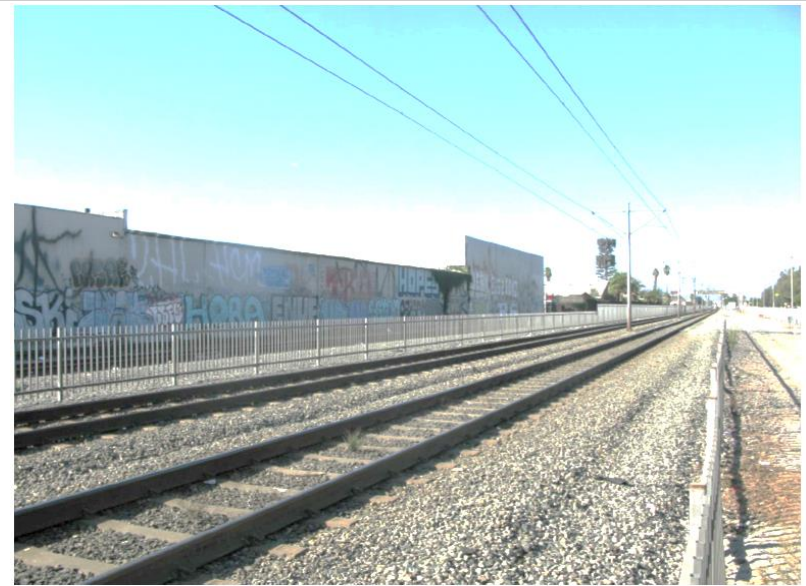
Adjacent Property Graffiti
