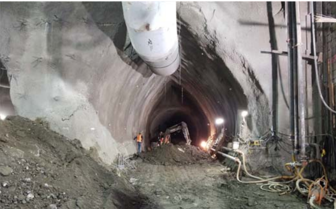
SEM Cavern right drift excavation
