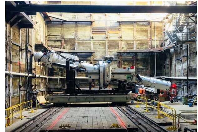
TBM Screw Conveyor at Wilshire/La Brea Station
