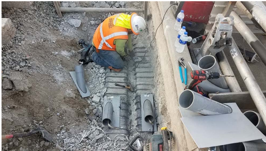
Modifying Existing Duct Bank
