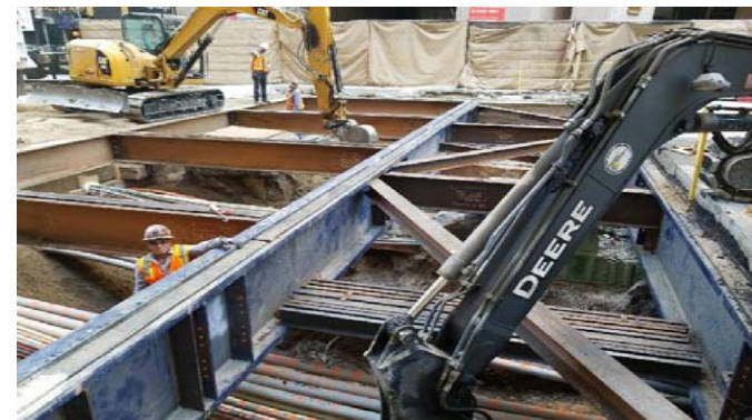
Excavation around utilities and deck beams on Flower Street
