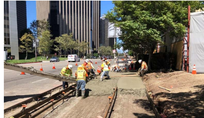
Concrete Placement for Staging Area Driveway in Century City
