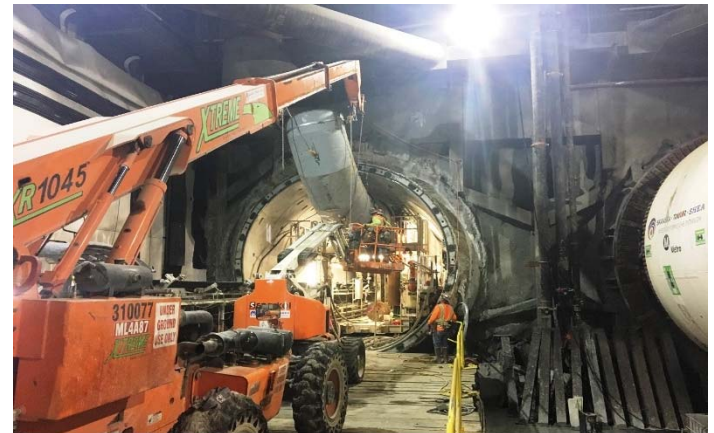
Wilshire/La Brea Station – Hanging Ventilation at Tunnel Heading
