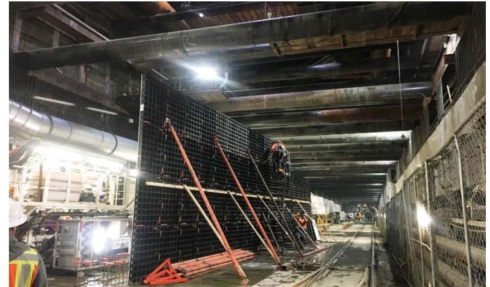
Wilshire/La Brea Station – Setting forms for Interior Walls
