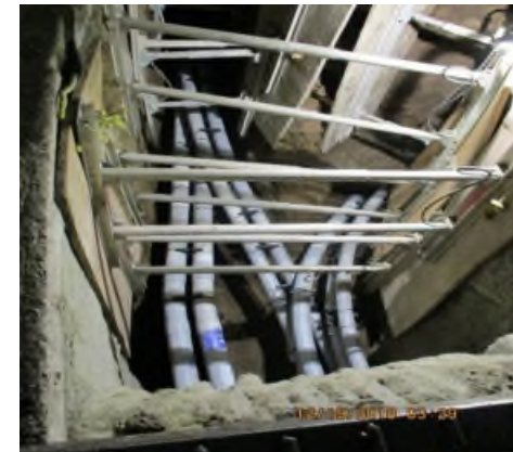
Conduit Installation on Wilshire Blvd.
