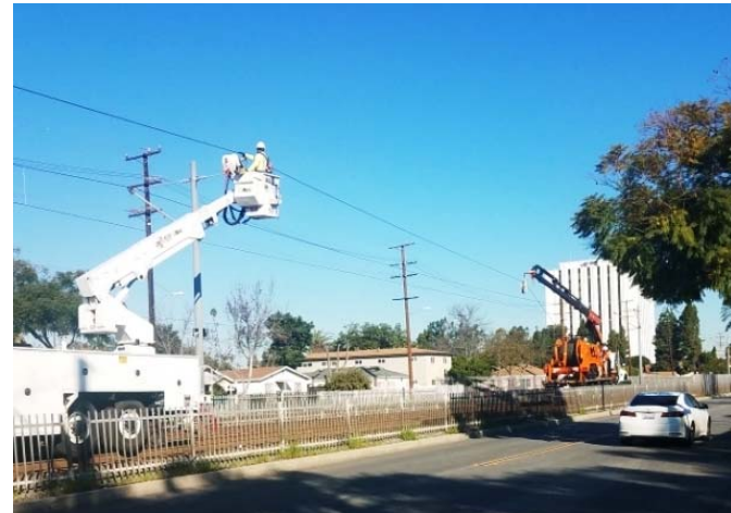
Overhead Catenary System Demolition
