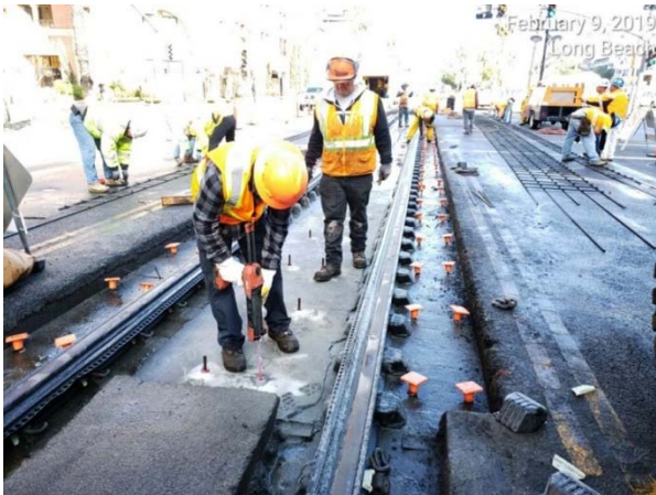
Rail Replacement at Long Beach
