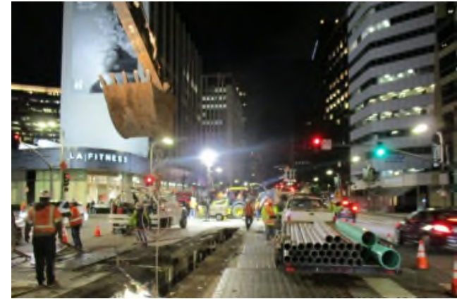
LADWP Water Pipe, Valve and T-Section Installation
