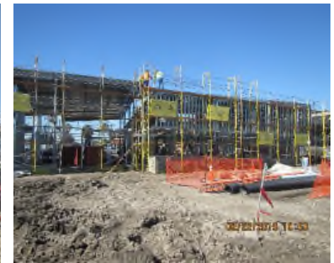
Framing for Customer Service Building
