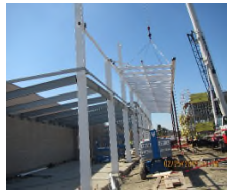
Structural Steel Installation for Mobility Hub
