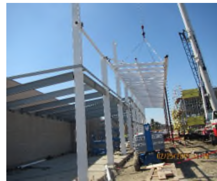
Structural Steel Installation for Mobility Hub
