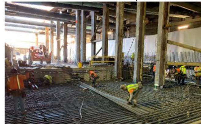
Rebar and MEP installation at 1st/Alameda Wye
