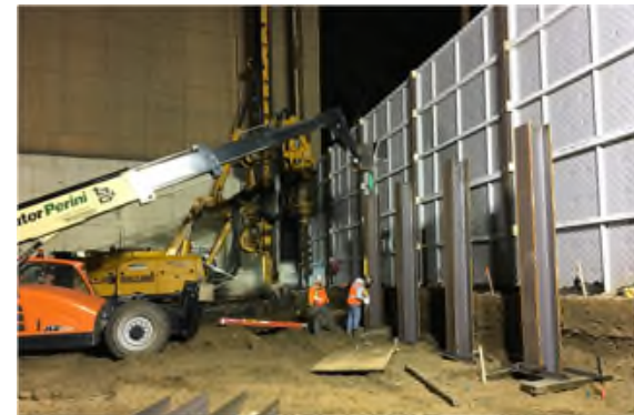
Muck Bin Pile Installation
