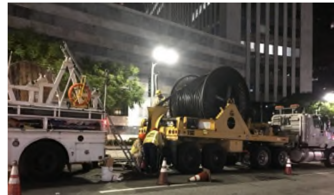
LADWP Cable Pulling
