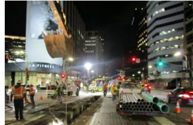
LADWP Water Pipe, Valve and T-Section Installation
