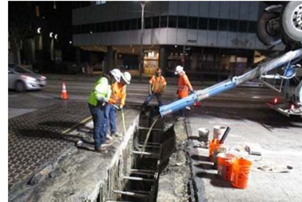
Slurry Backfilling Laterals on Wilshire Blvd.
