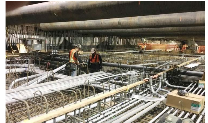
Installation of Conduit at Wilshire/La Brea Station
