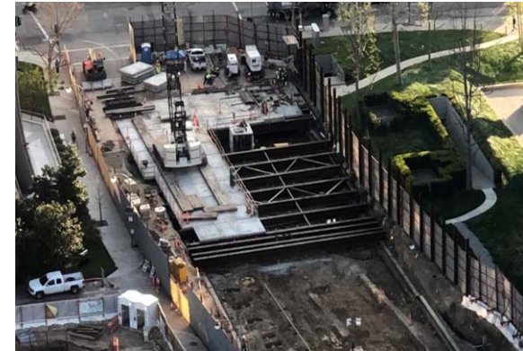
TBM Launch Box Overview
