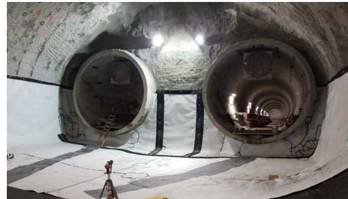
HDPE installation at SEM Cavern headwall
