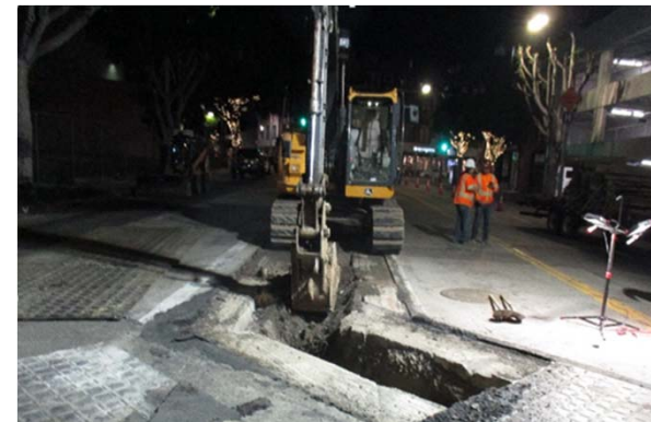
Water Line Excavation and Potholing
