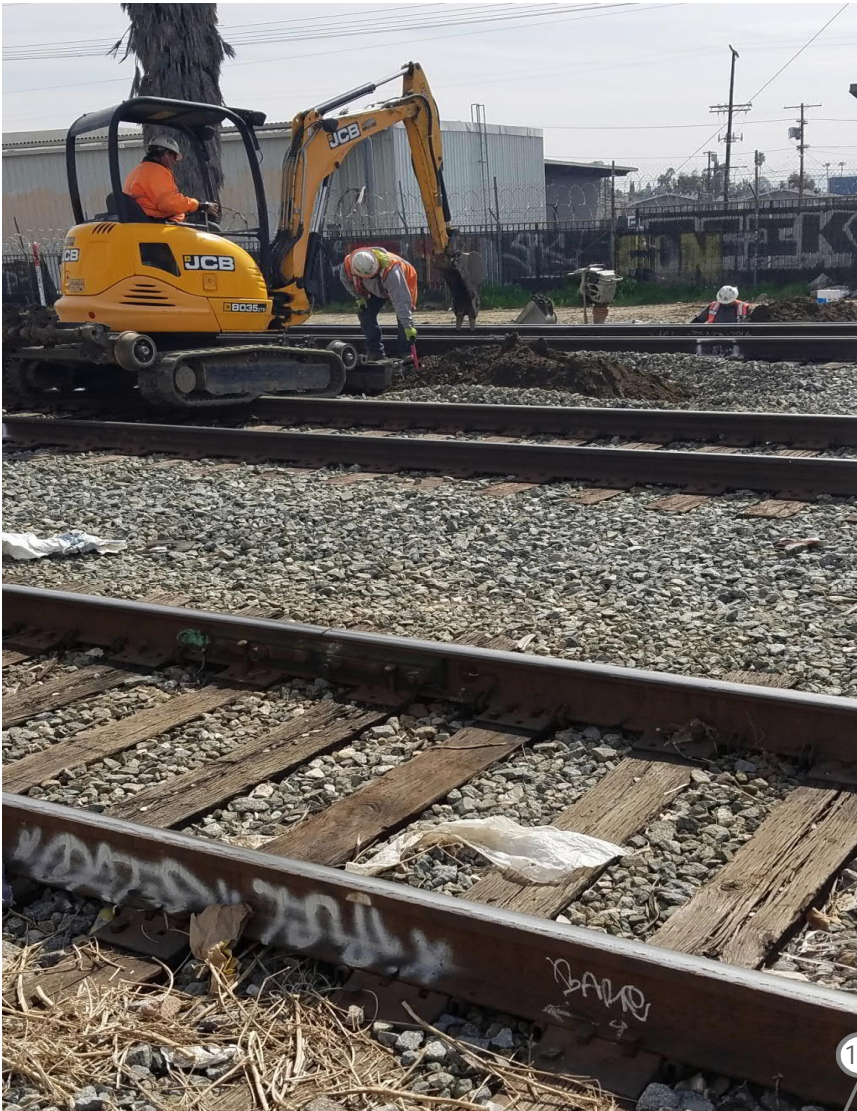
Photos: 1 (left): Signal trenching prior to turnout replacement at CP Woodman. 2 (right): Pre-built #10 turnout at CP Woodman.
