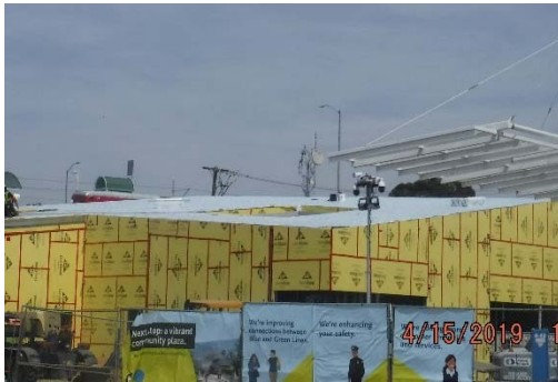
Exterior sheathing at Customer Service Building
