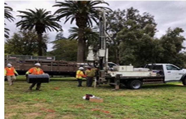
Geotechnical Investigations at VA Hospital for Tail Track Exit Shaft
