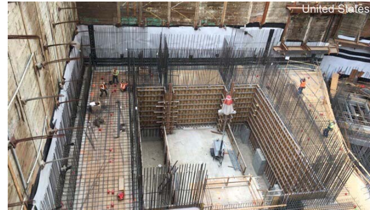
Rebar installation at Ancillary Level of Grand Av Arts/Bunker Hill Station
