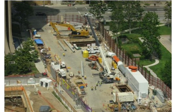
TBM Launch Box Overview in Century City
