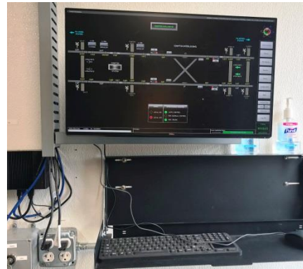
New Compton Interlocking Local Control Panel (LCP)
