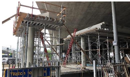
Formwork @ Blue Line Platform/Mezzanine
