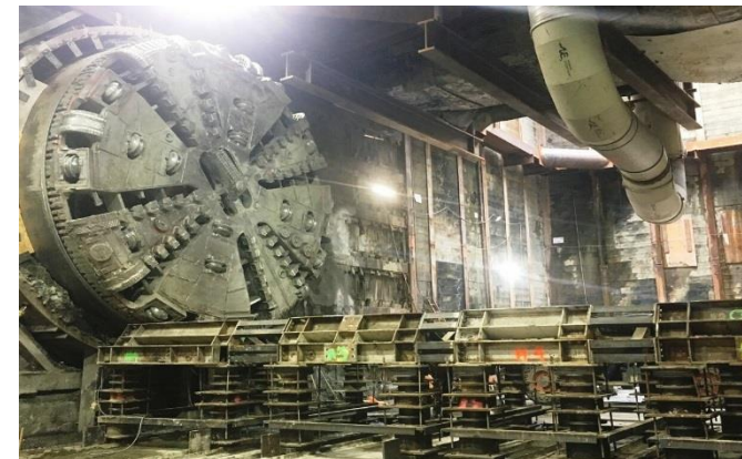
Preparations for Retrieval of TBM #1 at Wilshire/Western
