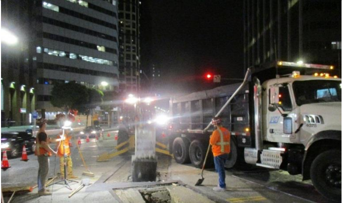
Main Line A Excavation and Potholing
