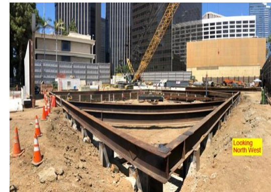
Tunnel Shaft Excavation in Century City
