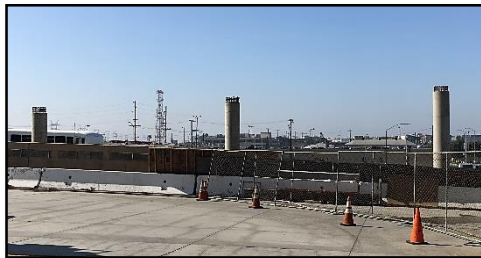
Pedestrian Walkway Columns
