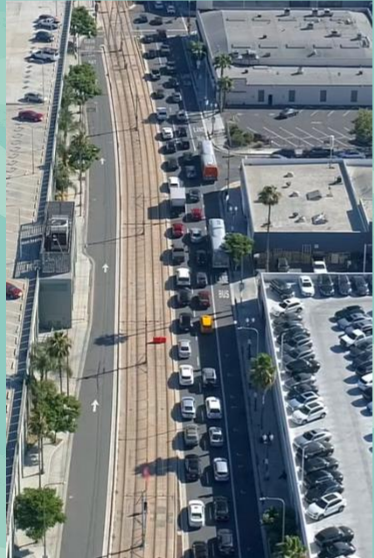
Flower St Bus Only Lane near LATTTC/Ortho Institute Station
