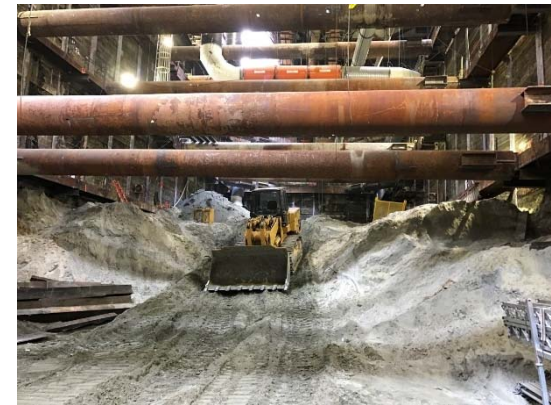
TBM Launch Box Excavation in Century City
