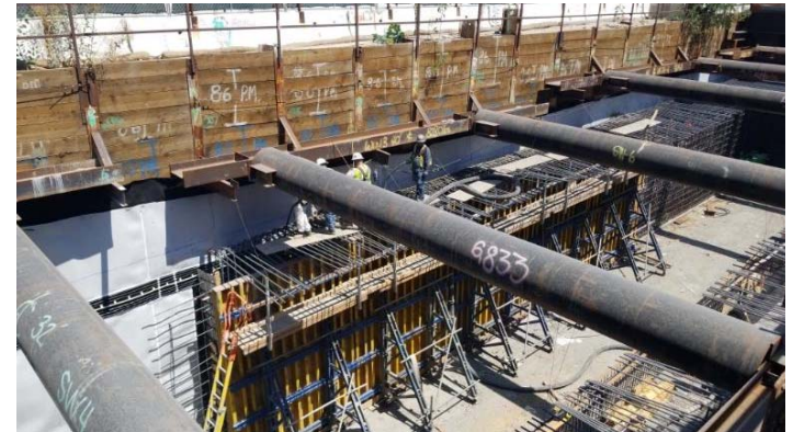
1st Street Cut/Cover Walls pour preparation
