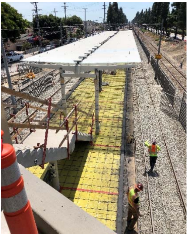
Blue Line Platform Work
