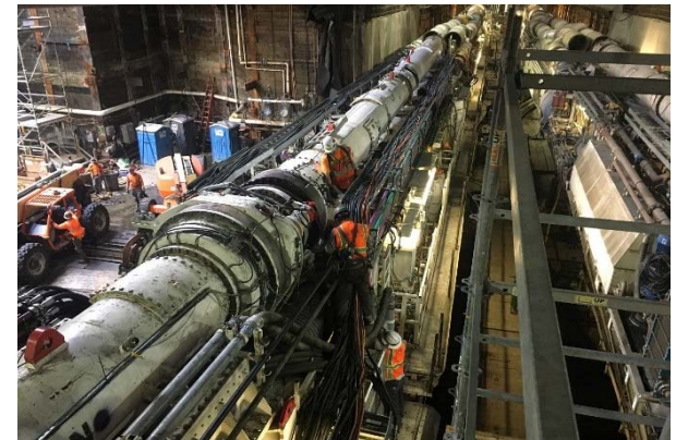
TBM Assembly at Wilshire/La Brea Station
