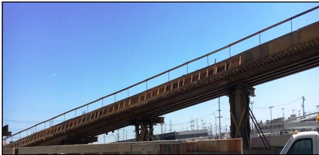
Pedestrian Walkway False work
