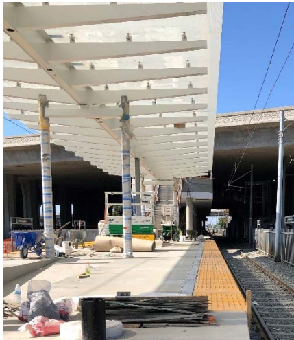
Blue Line Platform Work
