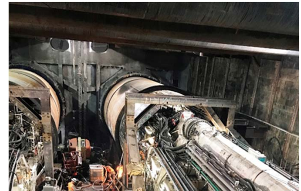
TBM Launch at Wilshire/La Brea Station
