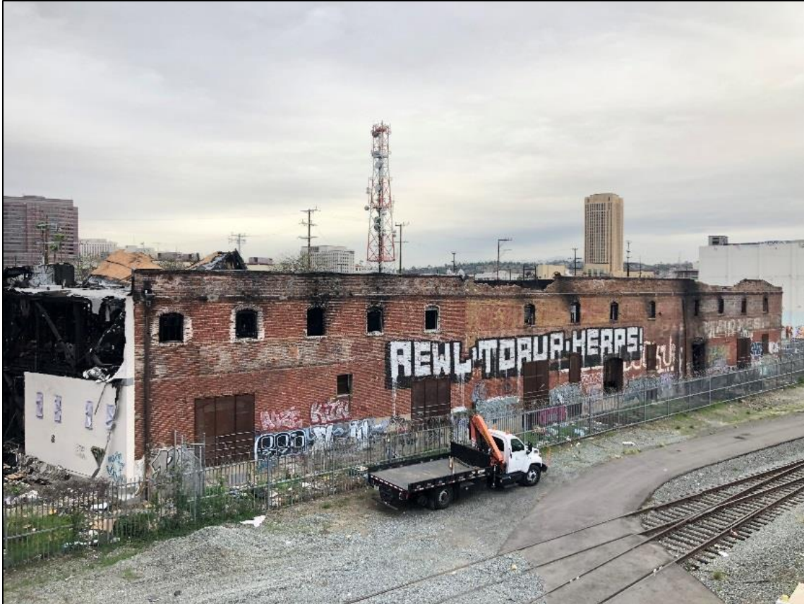
Figure 10. Citizens Warehouse/Lysle Storage Company (Pickle Works). East elevation. Looking northwest. ICF: November, 2018.
