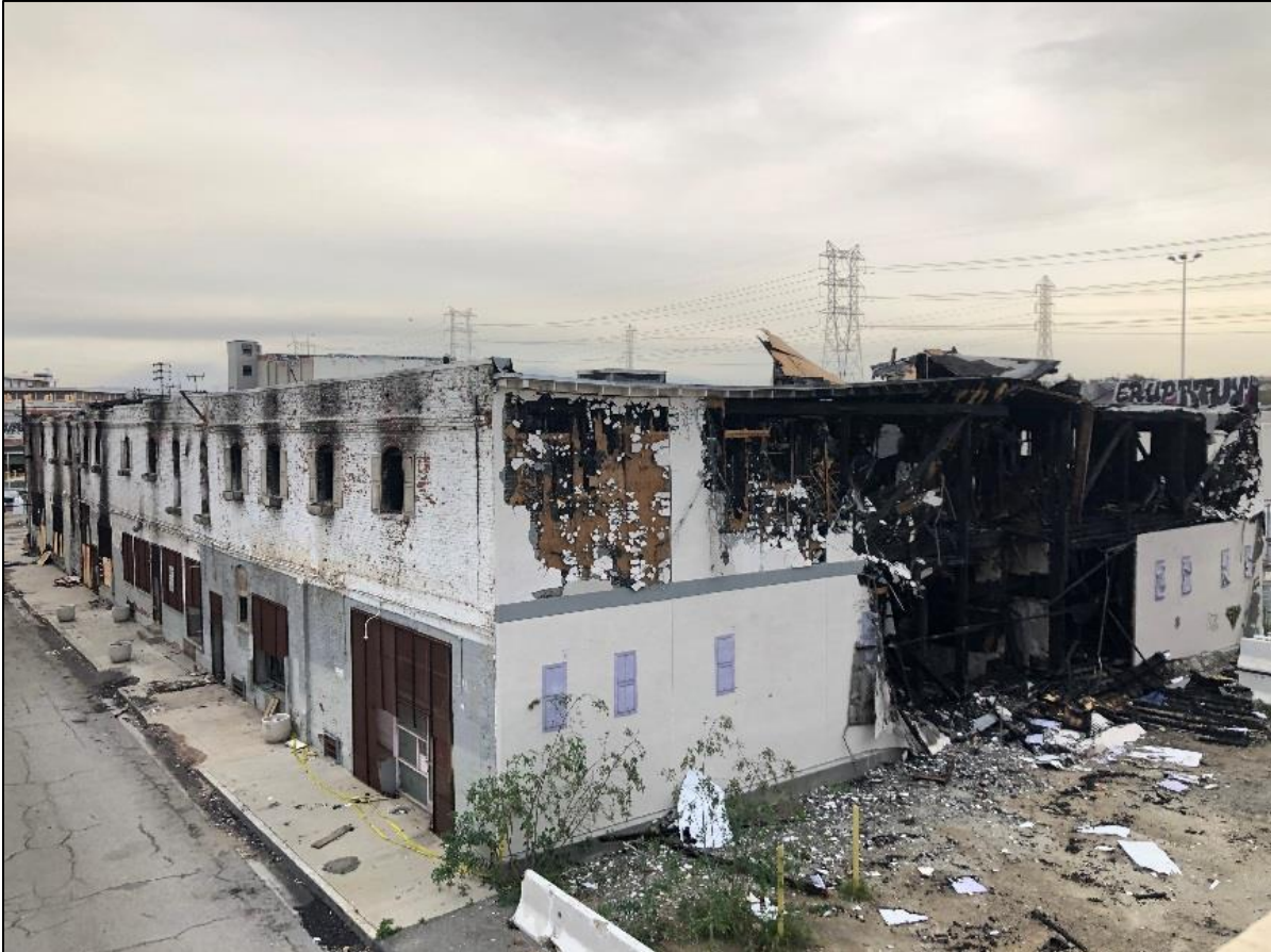
Figure 11. Citizens Warehouse/Lysle Storage Company (Pickle Works). West and south elevations. Looking northeast. ICF: November, 2018.
