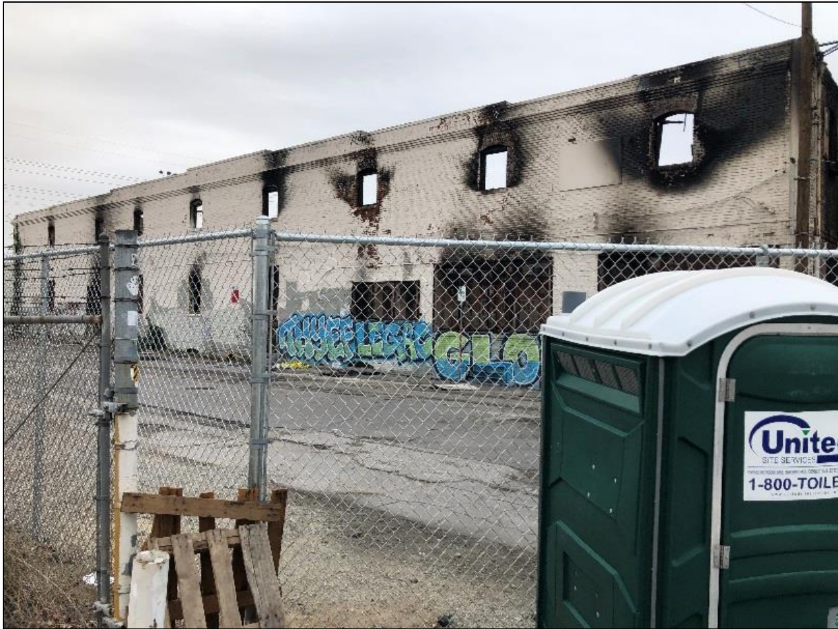
Figure 9. Citizens Warehouse/Lysle Storage Company (Pickle Works). North elevation. Looking southeast. ICF: November, 2018.
