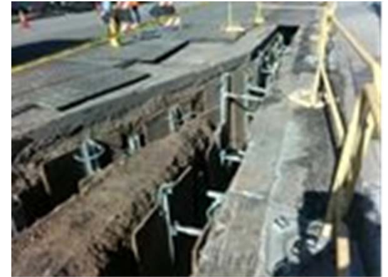
SCE Ductbank Trench Shoring
