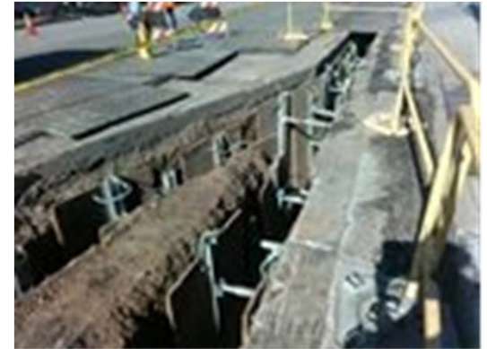
SCE Ductbank Trench Shoring
