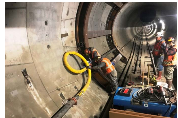
Excavation Preparation at Cross Passage 13
