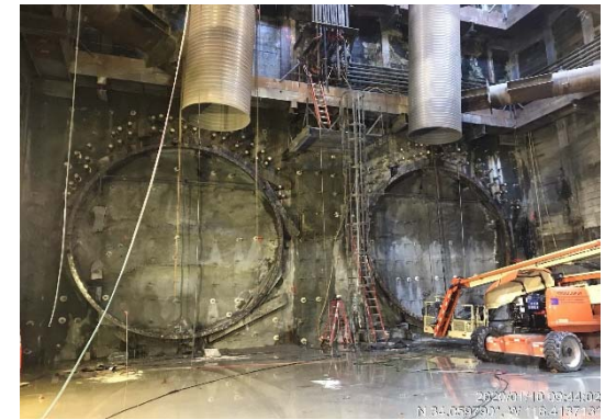
Tunnel Eyes at the TBM Launch Box in Century City
