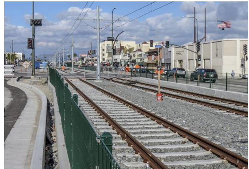
Trackwork and overhead catenary system – Crenshaw & 57 th
