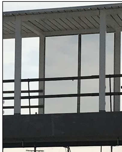
Interior panels initiated
