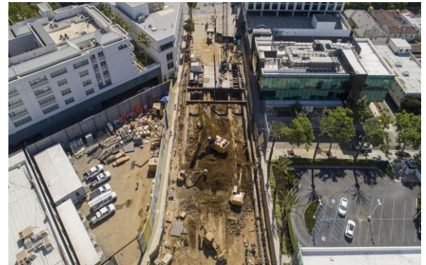
Street Decking Installation on Wilshire Boulevard
