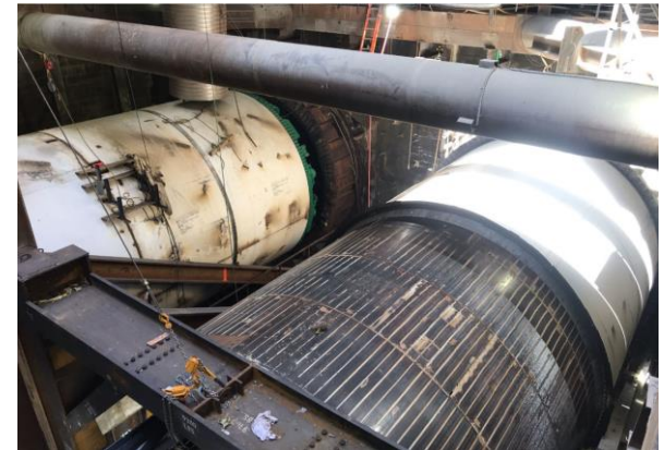
Launch of the first TBM in Century City
