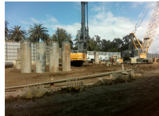
Pile Installation for TTES
