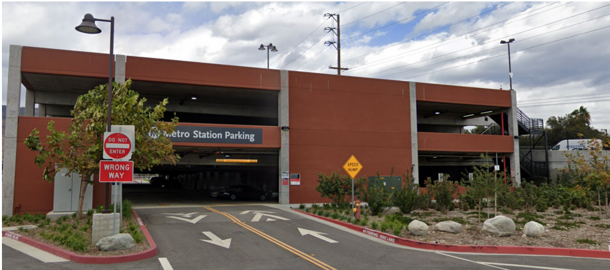
Figure 4.10.3 Irwindale Parking Garage (view from Jardine De Rosa off Irwindale Avenue)
