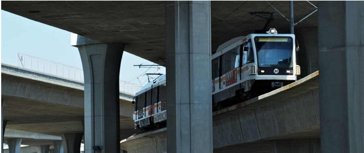
Figure 4.3.3 Metro C Line
